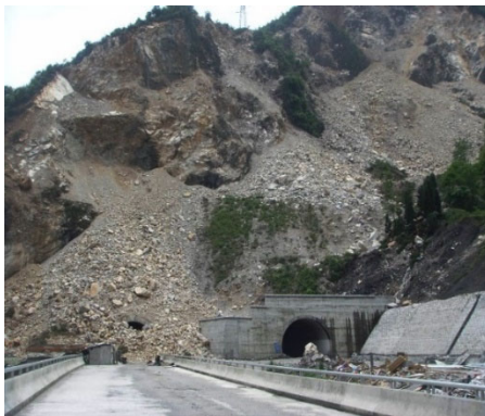
Invert slope damage at the entrance of Longdongzi Tunnel caused by Wenchuan Earthquake
